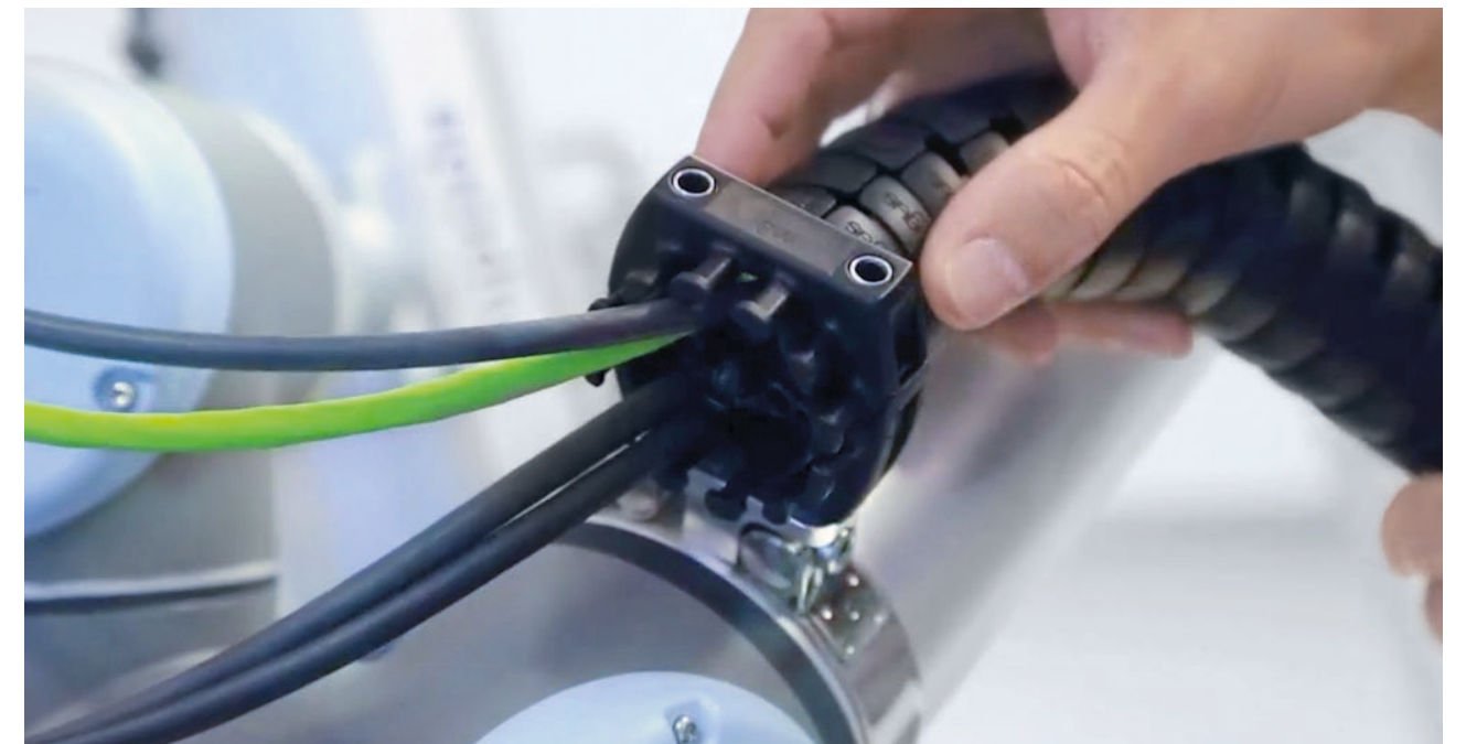
Fig. 18: Installation of a raceway (6)
